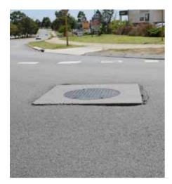
Steel utility covers can present a very slippery surface to a motorcycle or scooter.
