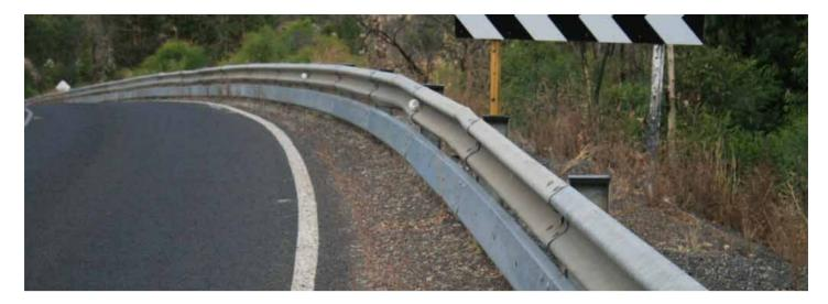
An example of additional protection added to a barrier to allow a rider to slide along the barrier and prevent colliding with a post in a crash.
