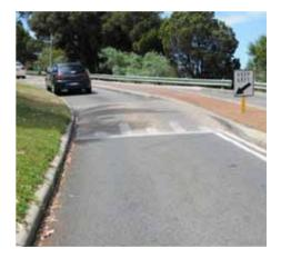
Speed humps located within and close to bends can present a serious hazard to motorcyclists.
