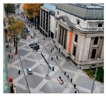
The above example, Exhibition Road in the heart of London, has removed all signage, lights, kerbing and pavements to create an environment where drivers take more care when travelling through the area.<sup>6</sup>
